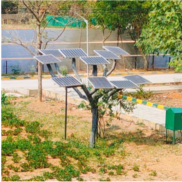
Fig 5: Solar Panel Installation on the field
