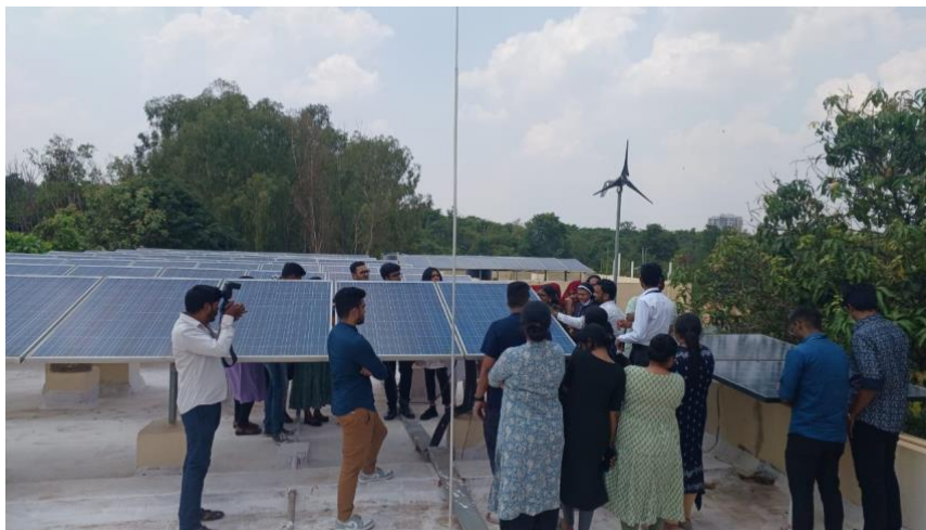
Fig 4: MGIRED faculties explaining about the Solar Panel Installation
